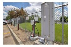
AUI installed four Leviton Electric Vehicle (EV) chargers at its Head Office in the fall of 2021. These chargers are level 2, meaning they can fill most EVs within five hours from empty.
